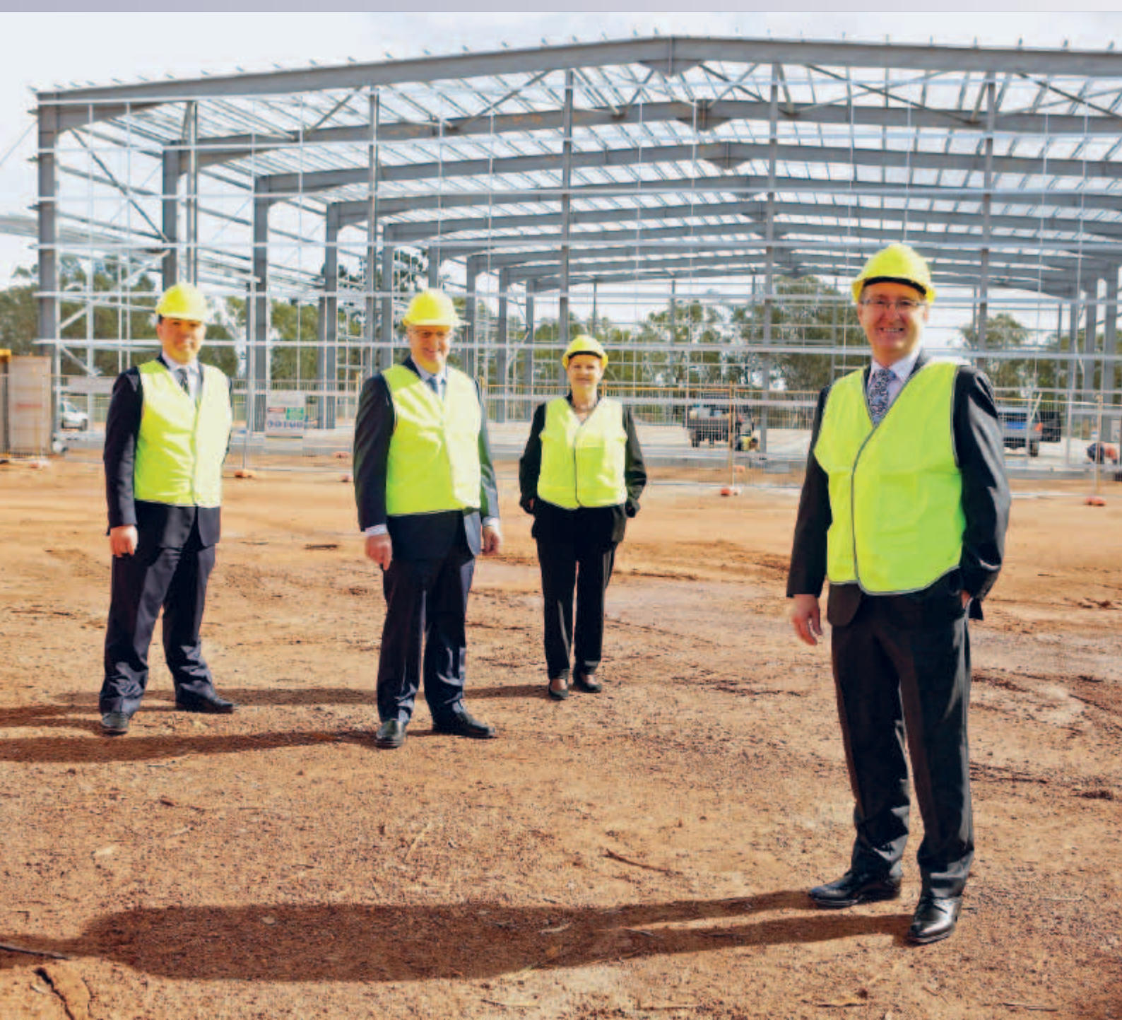
Commercial and Industrial Waste Sorting Facility under construction – June 2016
