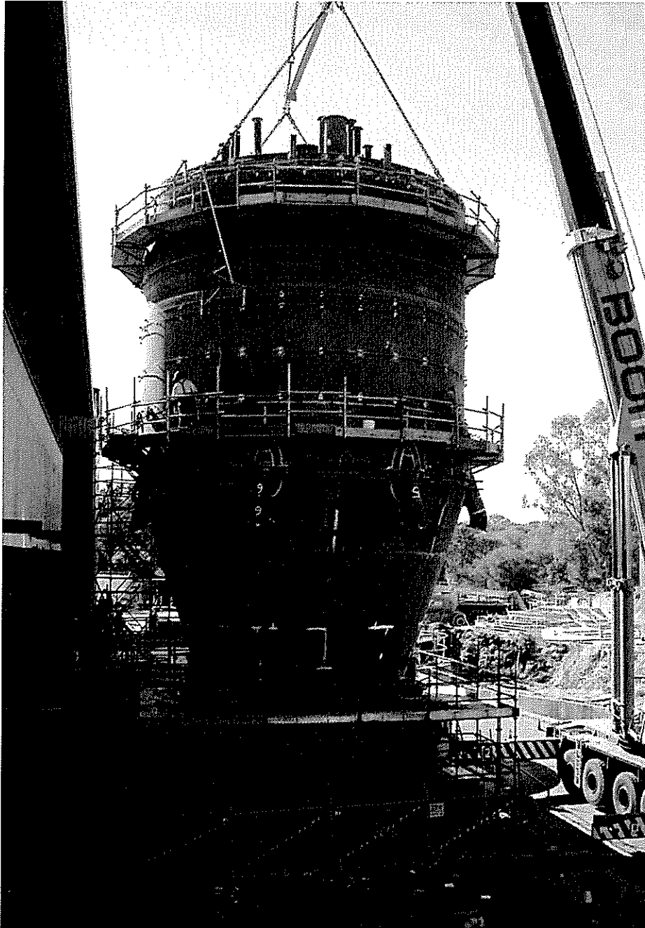
4. DiCOM vessel – all sections complete.
