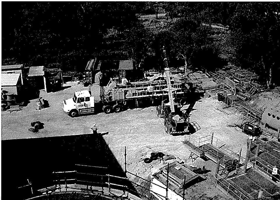
8. Yard at transfer station showing delivered equipment awaiting installation. This includes conveyor systems on truck waiting to be unloaded.
