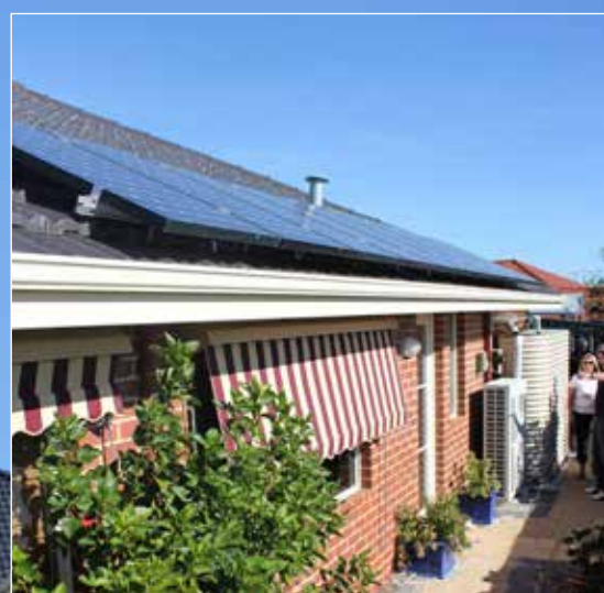
Image 10-F: The Eco House's summer savers – solar PV system, external awnings and water tank
