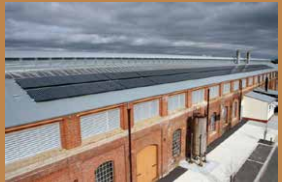
Image 13-B: Midland Foundry's 60kW solar PV system
