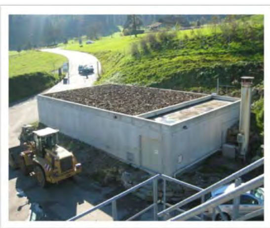
Figure 9 Example of a Biofilter
