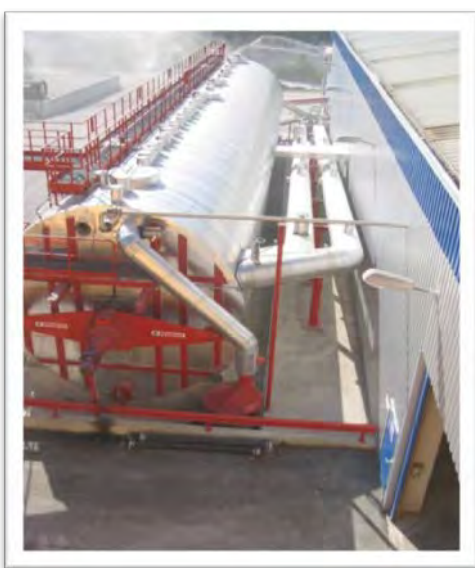
Figure 7 Example of a Horizontal Dry System Digester
