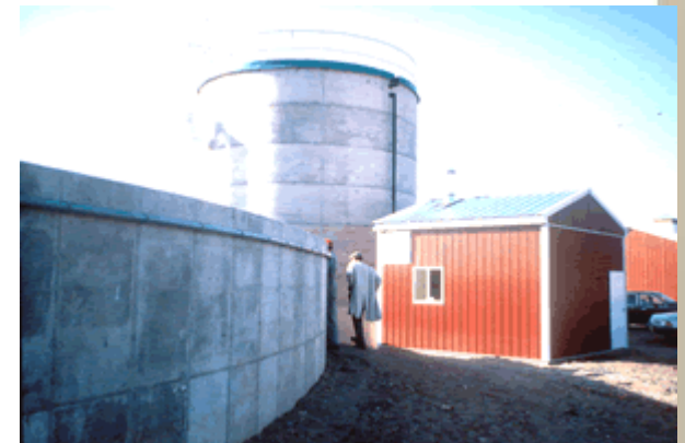
Complete mixed digester: (Cooperstown, NY: mesophilic or Thermophilic, manure 3 to 10 % Total solid)
