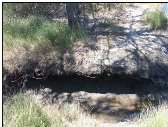
Erosion along drainage lines at Maylands Foreshore – City of Bayswater. Severe undercutting can be seen below the root zone (photo provided by NMCG).
