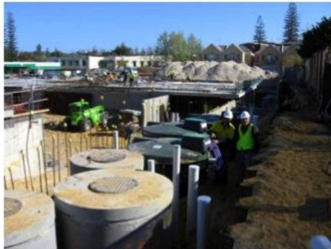
Figure 5: Photo of installation of wastewater recycling system at the Cottesloe - Peppermint Grove - Mosman Park Combined Library Source: http://thegroveprecinct.com/the-building/water-systems/#wastewater
