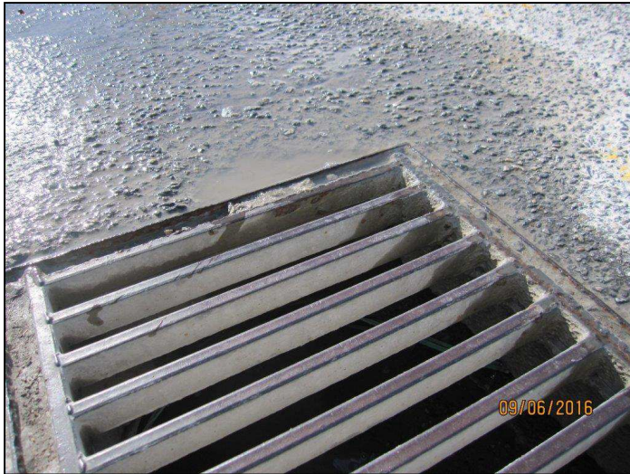
Photo 1: Cement running into Drain 3 on the corner of Wells and Irwin Streets (sub-catchment 4)
