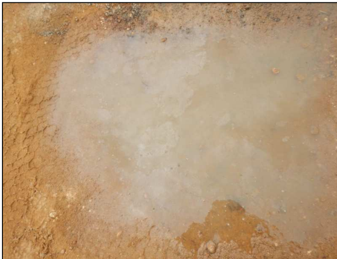
Photo 1: Cement running into Drain 3 on the corner of Wells and Irwin Streets (sub-catchment 4)
