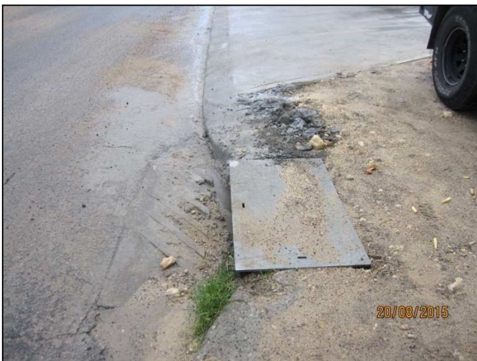
Photo 3: Site visit prior to sampling – cement and stone rubble around drain.
